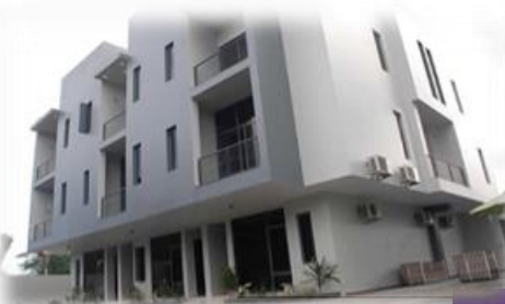
A 24-unit block of luxury 3-bedroom townhouses on Ojora Road, Ikoyi, Lagos, completed in June 2017 over 18 months.
