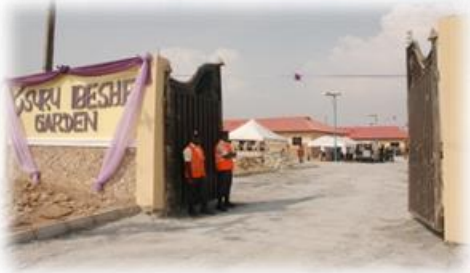
Completed in September 2012, this 26-unit low-cost housing project in Ibeshe Ikorodu, Lagos, was delivered in 6 months.
