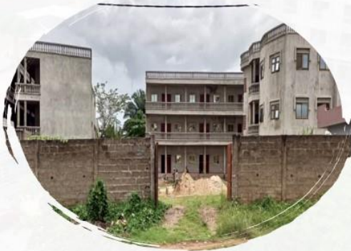
48 units of mixed development in Port Novo
